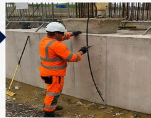
Precision injection restores monolithic integrity and prevents future ingress.
