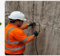
Precision injection restores monolithic integrity.
